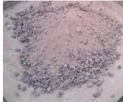
Fig 6.1 Mixing Of Concrete Raw Materials
