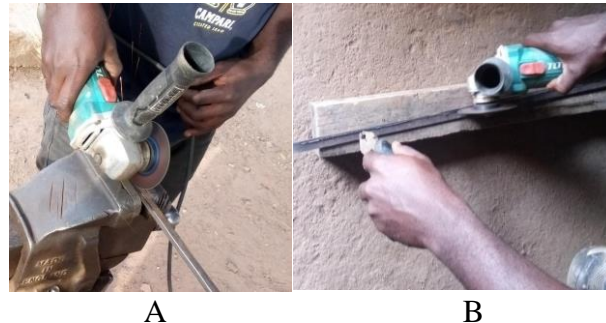
Figure 45: Cutting of metal into required sizes for frame using cutting machine (AB)
