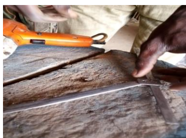
Figure 50: Aligning vertical and horizontal metal of the frame
