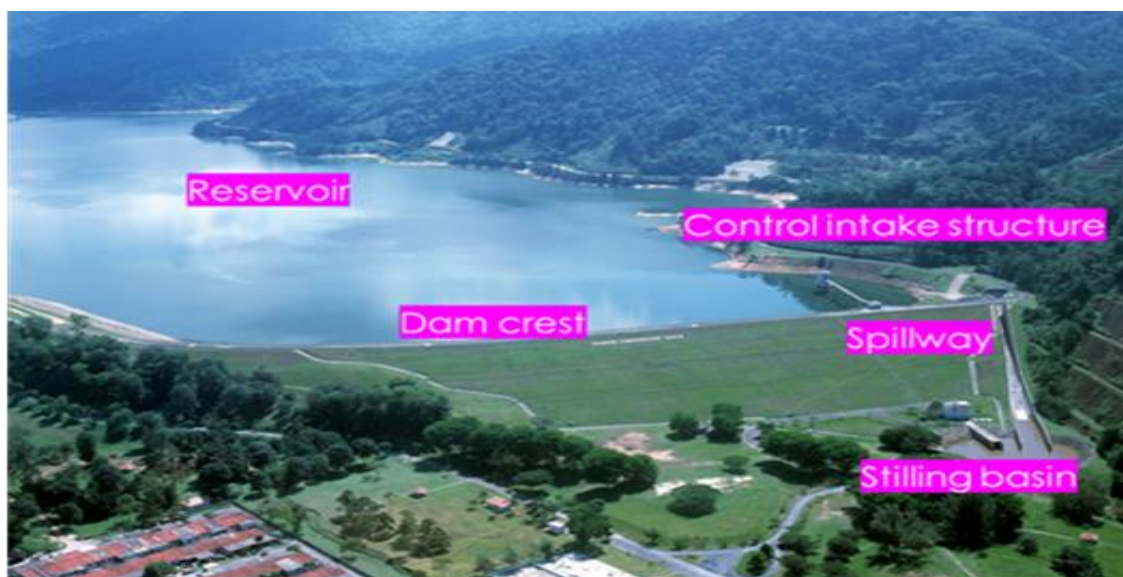
Fig. 2. The components of Batu Dam, Malaysia.
