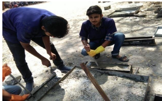
Figure 3.2 Compaction of prism mould
