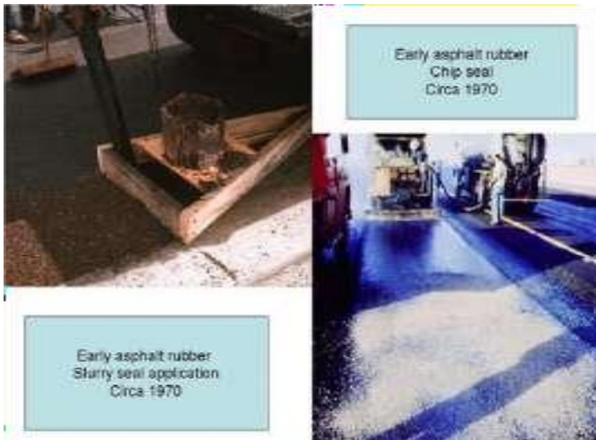
Figure 2- Rubberised bitumen applied as a slurry seal
