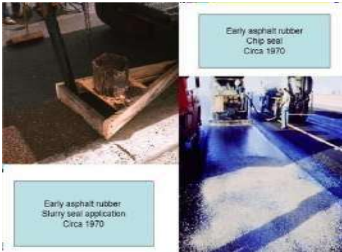
Figure 2- Rubberised bitumen applied as a slurry seal
