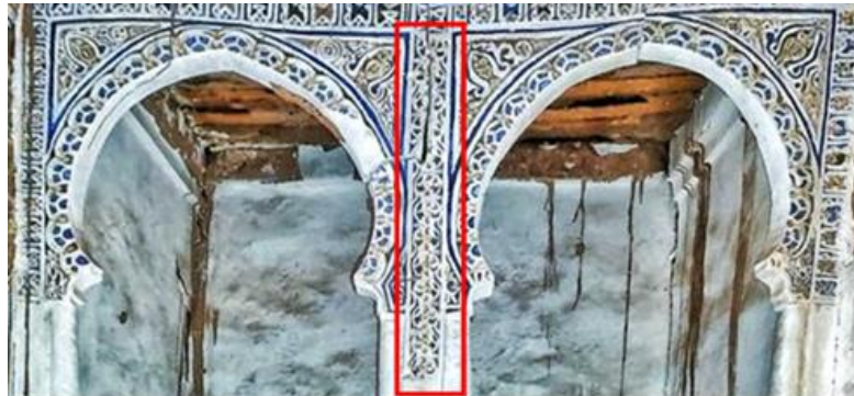
Figure N° 27. (The ribbon separating the two arches.)
