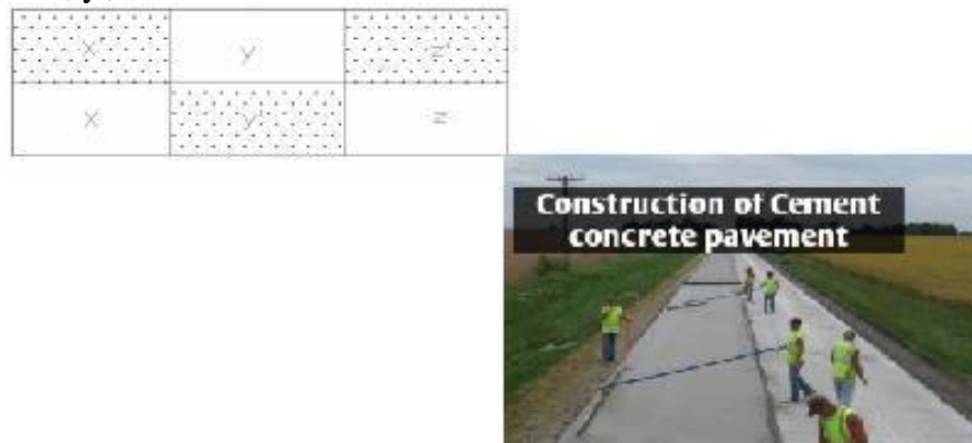
Fig. 1 illustrates the cement-based concrete construction process.
