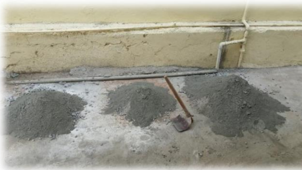
Fig: 3.4. concrete mixing progress
