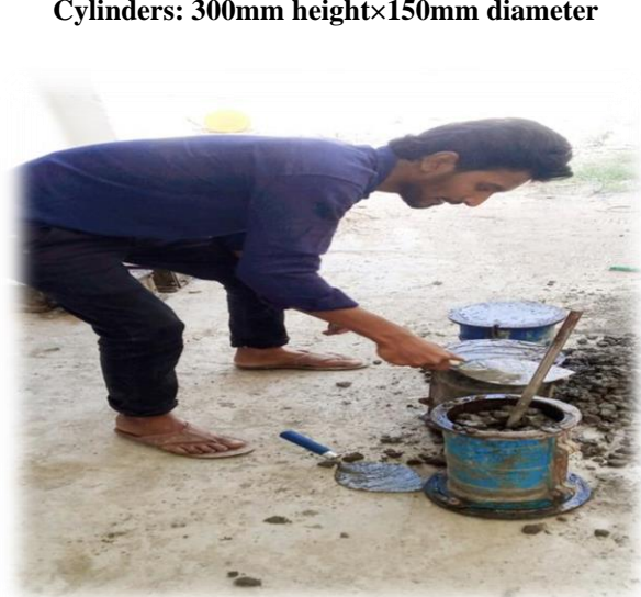
Fig:3.6 Casting and Compaction of Cylinders
