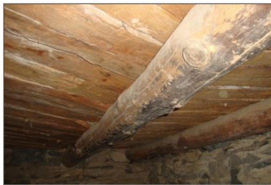
Image 7: The Flat Roof of the Lobby
