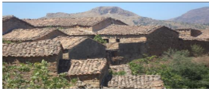
Image 3: Closely Packed and Aligned Houses
