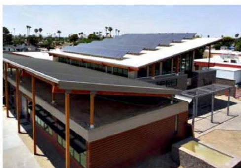
Form (1-1) Use of photovoltaic panels in schools
