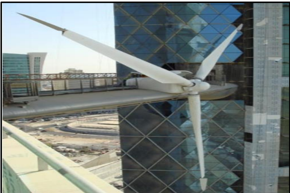
Fig 19. Barain WTC Wind Turbines with the Bridge
