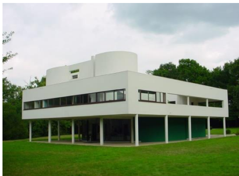
Image (18). Le Corbusier's method of demolishing the box building by raising the building on pillars and using strip windows to communicate between the inside and the outside / Wikipedia
