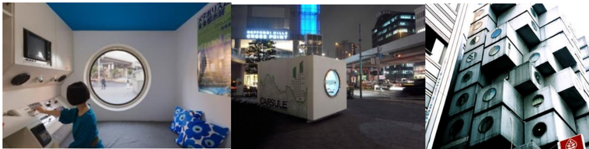
Image (11) Link 1. The capsule from inside and outside, which is Image (10). The facade prefabricated and transported by trucks and lifted to be fixed on the steel axle.
