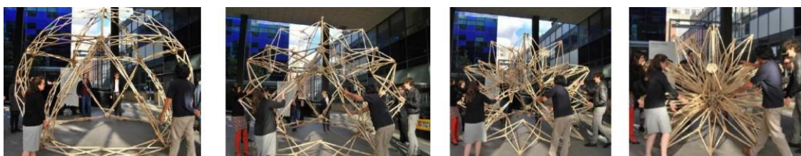
Image (7) A polyhedral dome with triangular units formed by several images (internet web)
