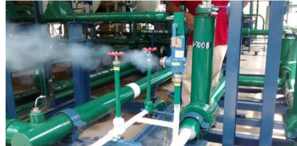
Fig. 4.5 Cryogenic pressure relief valve
