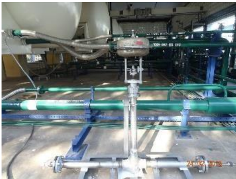
Fig. 4.3 Cryogenic globe valve
