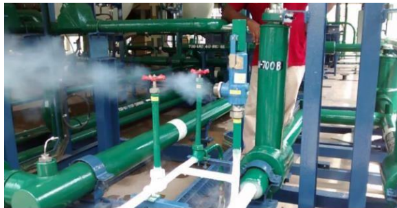
Fig. 2.1 Cryogenic PRV in operation at LSSF
