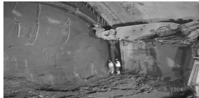
Figure 9: Installation of the forepoling tubes at the top heading of the station tunnel [7].
