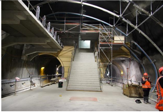
Figure 2: Using of NATM method for station construction
