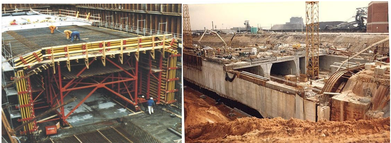
Figure 3: Some view of NATM construction method Fig. 4: Cut and cover construction method
