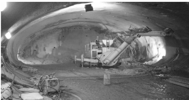
Figure 9: Installation of the forepoling tubes at the top heading of the station tunnel [7].
