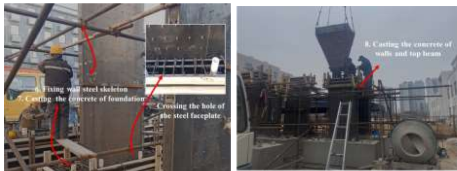
(c) Fixing wall skeleton and casting concrete of foundation
