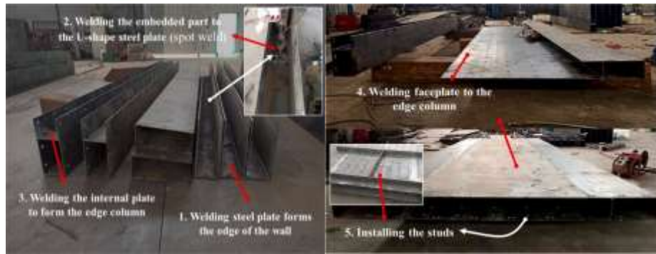
(a) Fabrication of edge column
