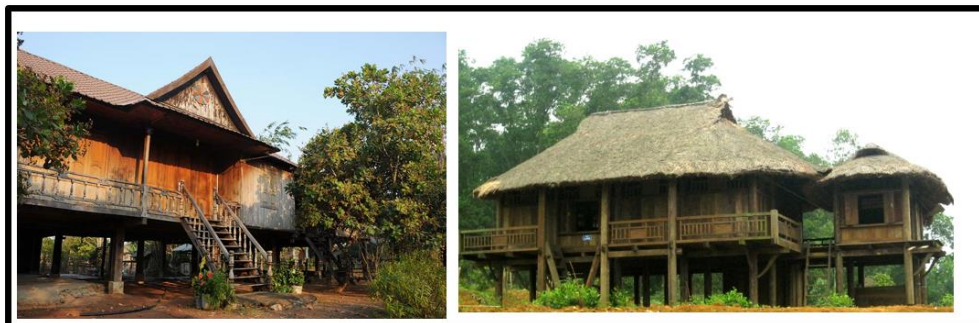
Fig. 6: Grass thatch roof of stilt houses in Laos
