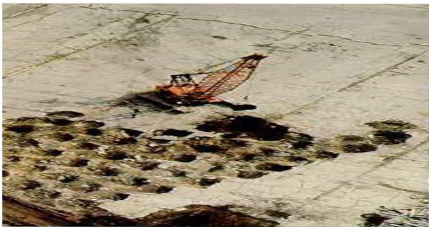
Fig.1 DYNAMIC COMPACTION
